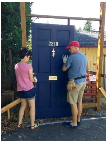
Maria and Oz installing the first door.
