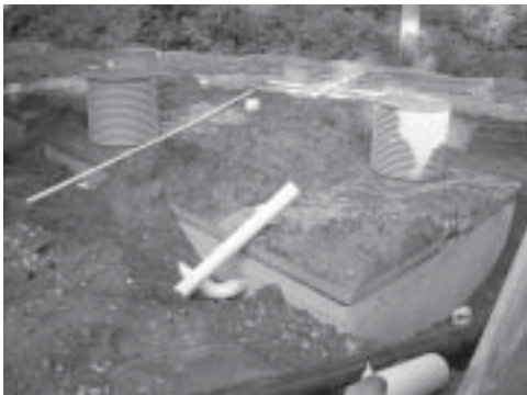
Septic tanks, where solids go.
