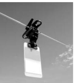
A Bird Mark flight diverter, similar to the models which will soon replace the old ones along Portage's power lines. A new model will include UV light in the flapper area to alert the birds at night.
