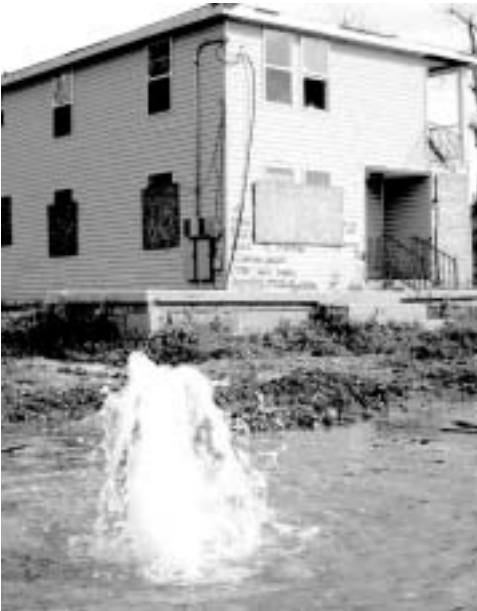
A broken water main outside of house in lower Ninth Ward. The City now loses more water than it uses due to damaged and faulty pipes. Spray paint left by search and rescue after Katrina or Rita. Photo by Logan Price, Feb 07.
