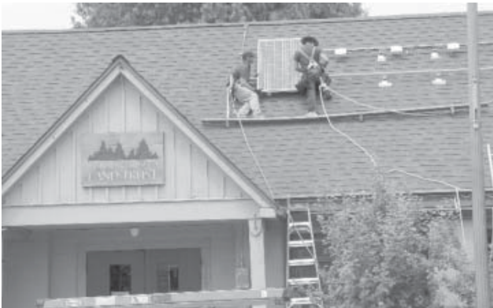
Workers begin installation of a 1.8 kW grid-tied solar system on the roof of the Vashon-Maury Island Land Trust building, photo by Dan Schueler.
