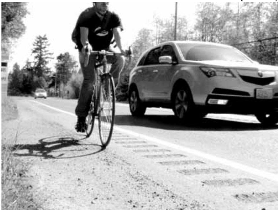
Rumble Strips already etched into the main road north of Town.
